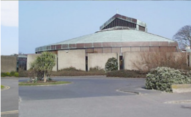
Saint Fintan's Church designed by the well known architect Andy Devane of the firm of Robinson Keefe and Devane, is a copper roofed, fan shaped church using textured concrete is one of the few modern churches of any quality in Dublin.
