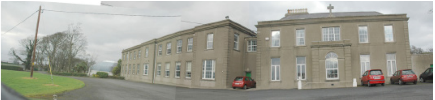
Much altered and extended Santa Sabina, somewhat overpowered by the 20th century secondary school and especially the more recent sports hall.
